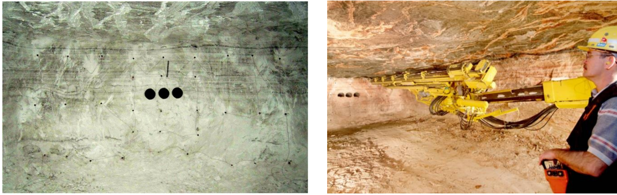
Figure 12: Transferred blast design on site (left and right) (source K+S)
